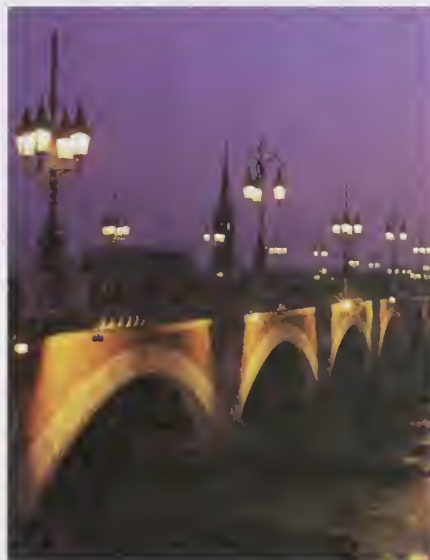
The Pont de Pierre bridge over the Garonne River, Bordeaux, Fr.
